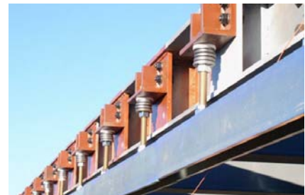
Figure 12 Top Shoe Detail.
