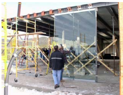
Figure 13 Panel Installation.
