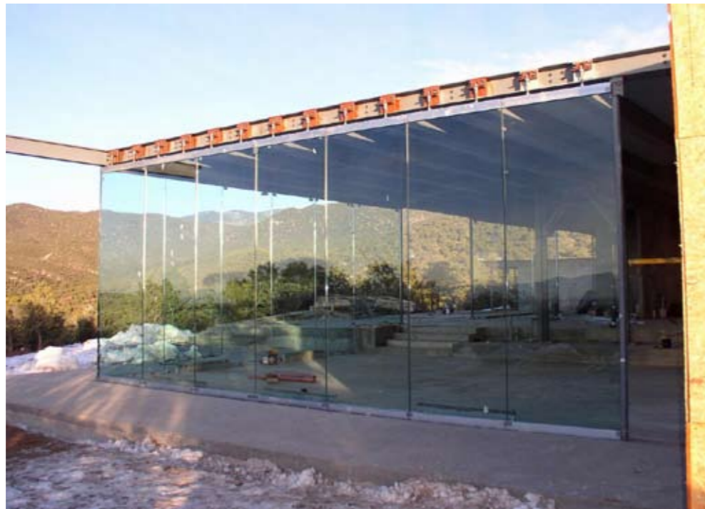
图例14 玻璃板安装完毕后 Figure 14 Completed Installation
